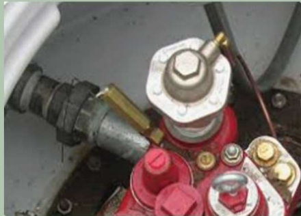
Leak Detection failure
